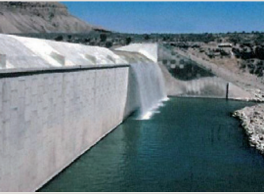
Taylor Draw dam on the White River, Colorado, USA
