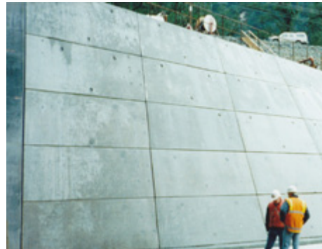
Manapouri second tailrace tunnel, New Zealand
