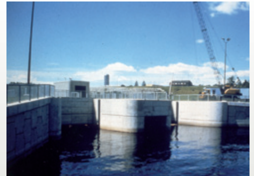
Allard dam, Canada
